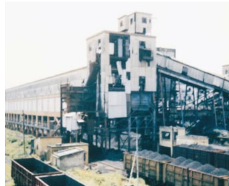
Through a recently completed agreement with USAID-India, FETC supported demonstration of a U.S. advanced coal cleaning technology at the commercial Bilaspur Coal Washery in Madhya Pradesh. This 2.5-million-ton/yr washery is being built through a joint venture among Spectrum Technologies of New York, CLI Corporation of Pennsylvania, and Bombay Suburban Electricity Supply of India. Additional site-specific cost-benefit studies have been conducted to support establishment of other coal beneficiation plants in India with U.S. partners.
