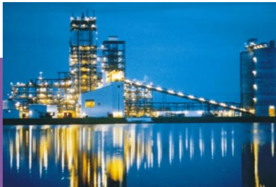
The Tampa Electric IGCC system, built as a greenfield site, is one of the cleanest and most efficient coal-fired powerplants in the world.
