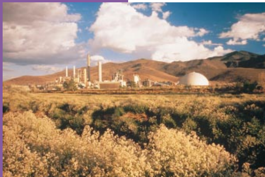
The third IGCC plant to become operational in the United States, the 100-MW Sierra Pacific Piñon Pine project near Reno, Nevada, demonstrates a KRW air-blown gasifier with in-bed sulfur capture, advanced hot-gas cleanup, and General Electric power generation. With an anticipated efficiency of over 43%, the plant will deliver more efficient, less costly, and cleaner electricity.
