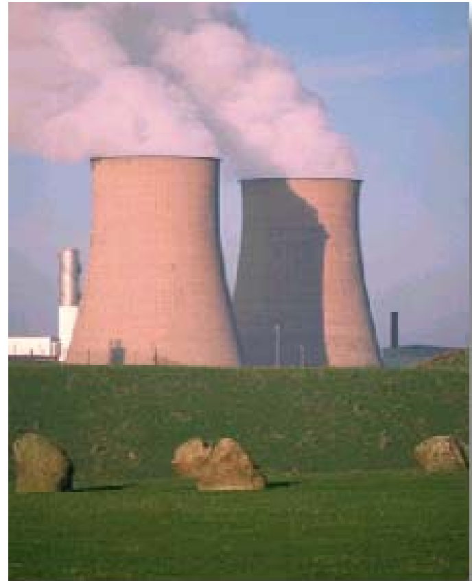
Power Plant Cooling Towers
