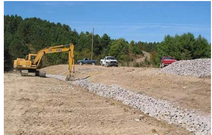
Installation of passive treatment limestone channel
