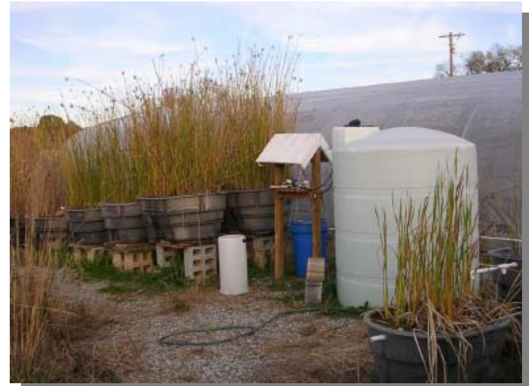
Photo of detention basin, pump house, and pilot-scale CWTS designed for ash basin waters
