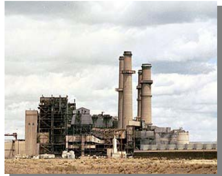
1,800 MW San Juan Generating Station (SJGS)
