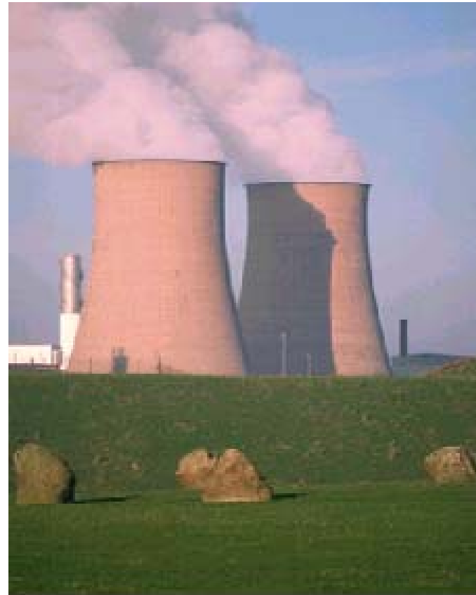
Power Plant Cooling Towers
