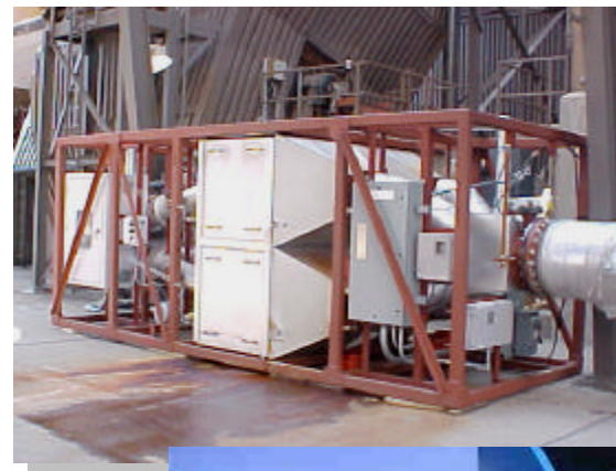
URS Pilot-Scale Catalyst Unit
