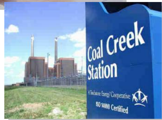
Great River Energy's Coal Creek Station, North Dakota
