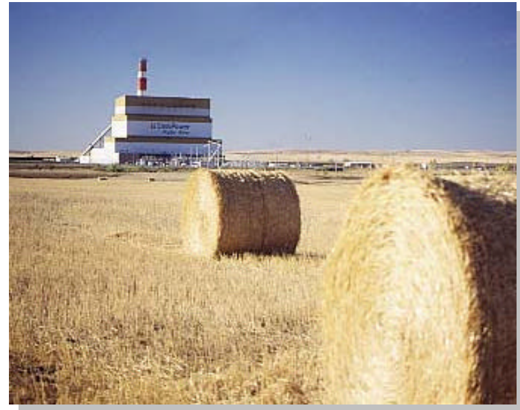
SaskPower's 562-MW Lignite-Fired Poplar River Power Plant
