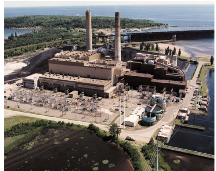
We Energies Presque Isle Power Plant
