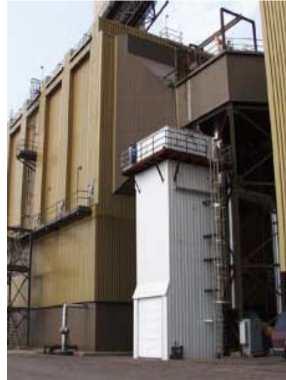
AHPC Slipstream Test Unit at Big Stone Power Plant
