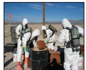
NTS F&R staff collects and places the neutralized nitric acid in 55-gallon drums for disposal.
