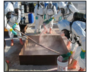
Members of NTS F&R release a neutralizing agent into the nitric acid.
