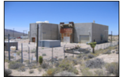
The Pluto Disassembly Facility will be investigated in Corrective Action Unit 117.
