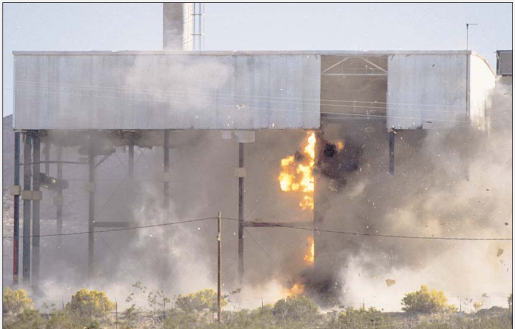
Below: Stripping away sheet metal and concrete walls leaves only the structural supports and reduces the amount of explosives required to bring down the structure. At right: The Controlled Explosive Demolition of a high bay structure at R-MAD.
