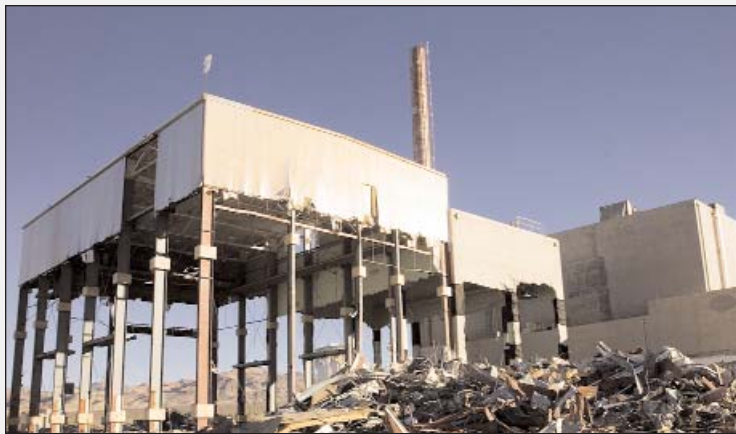
Below: Stripping away sheet metal and concrete walls leaves only the structural supports and reduces the amount of explosives required to bring down the structure. At right: The Controlled Explosive Demolition of a high bay structure at R-MAD.
