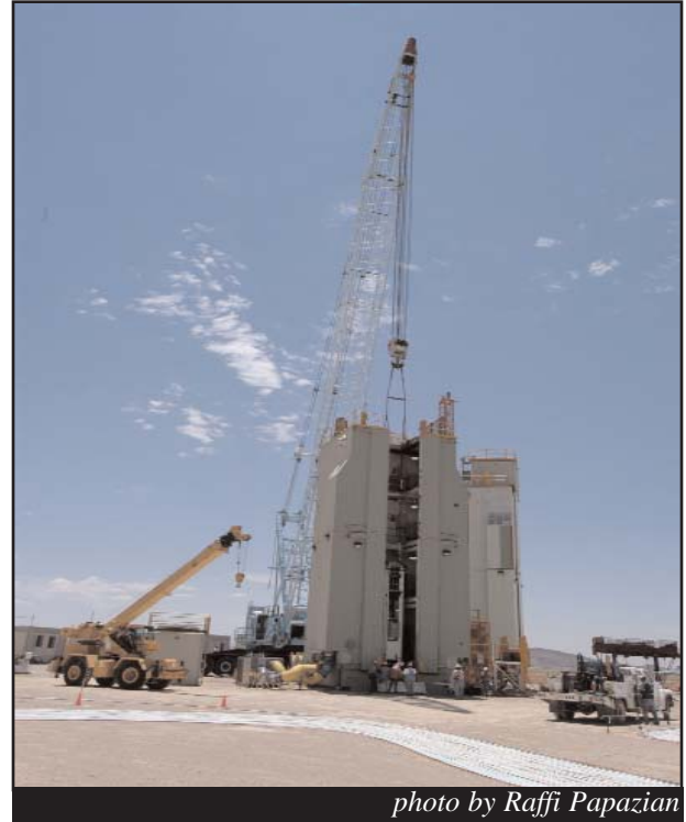
The Unicorn rack that will contain the experiment is placed in the Unicorn tower by the nuclear certified crane, "Big Blue." The tower for the Unicorn confirmatory, Centaur Experiment, is seen in the background.
