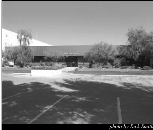
The B-2 building prior to demolition.
