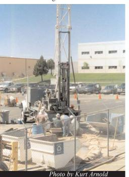
Bechtel Nevada's construction department uses a drill rig at the North Las Vegas facility to drill a well pair (one shallow and one deep) to monitor groundwater levels. Data gathered from the wells will assist in determining why groundwater is rising at the North Las Vegas facility.
