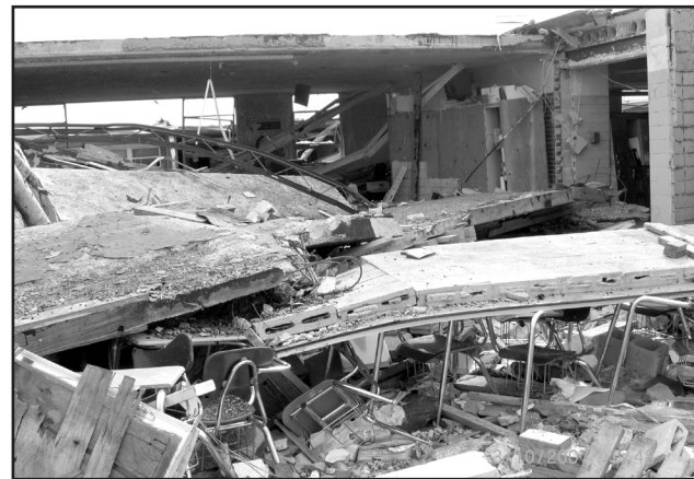
Figure 1-2. Destroyed tornado refuge area at Enterprise High School, Enterprise, Alabama (2007)
