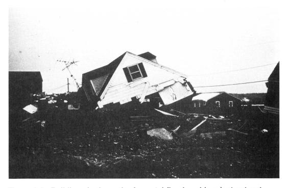
Figure 6-6: Buildings in the path of coastal floods seldom just get wet. Erosion worsens flooding as well as causing physical damage. Source: Jon Kusler.
