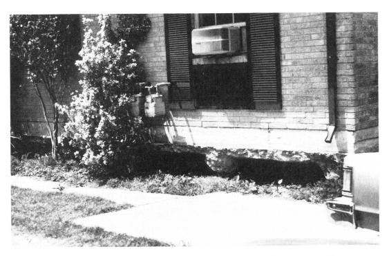
Figure 9-3. Subsidence on organic soils has resulted in structural damage to this house in New Orleans. Source: B. Cox.
