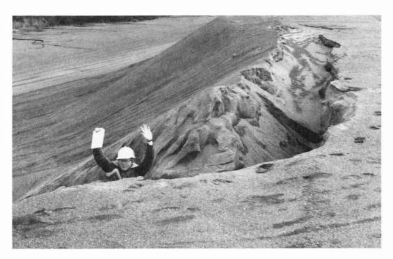
Figure 5-5. Routine dam inspection is a necessary part of a dam safety program. This rather dramatic erosion problem was identified during a routine inspection. Source: Minnesota Dept. of Natural Resources.
