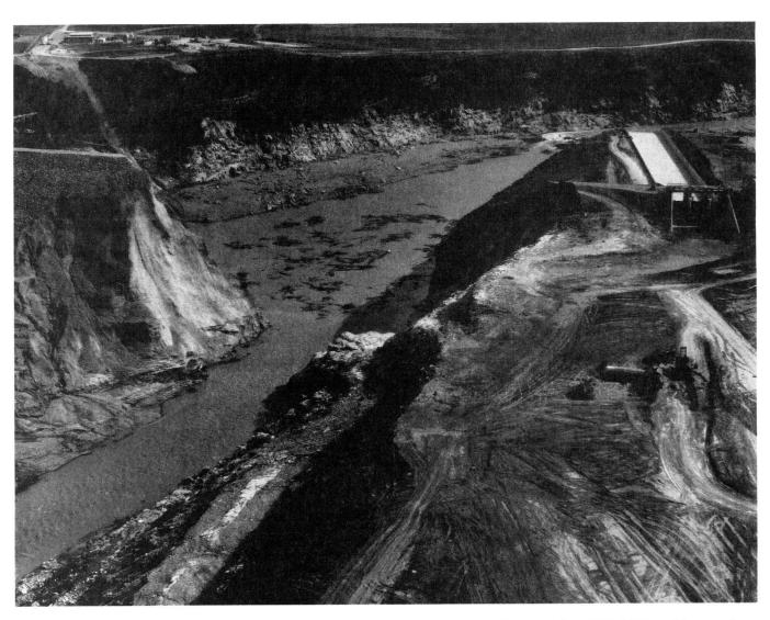
Figure 5-1. The Teton Dam, a Bureau of Reclamation project, collapsed in 1976 killing 11 people and causing millions of dollars in damages. The dam's collapse illustrated, once again, that structural solutions to flood problems are not without inherent risks.
