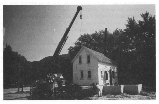
Figure 4-3. House behind levee in Soldier's Grove, Wisconsin being elevated after severe flooding in 1978. Source: T. Hirsch.
