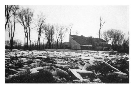
Figure 10-5. This house has been protected from flood and ice damage by being elevated on fill. Source: Mary Fran Myers.
