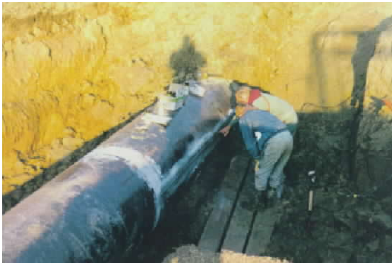
Magnetic Particle Inspection for Cracking
