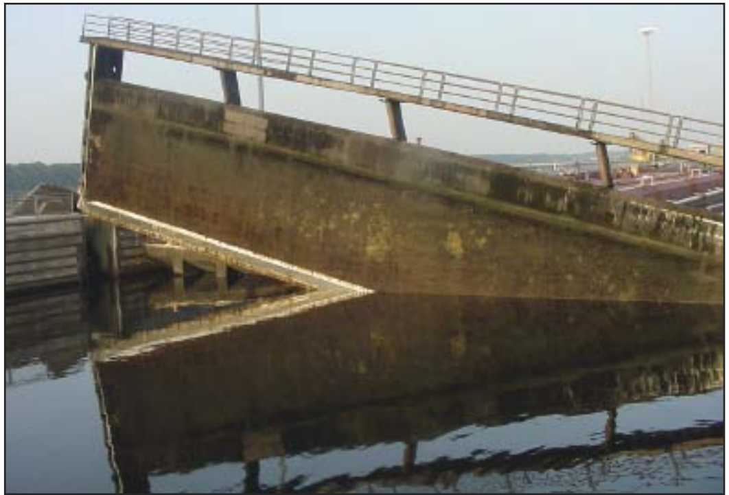
Figure 2: Wilson Lock/Dam upper main lock gate lifted from its track. USCG photo by CW03 Tim Smith.
