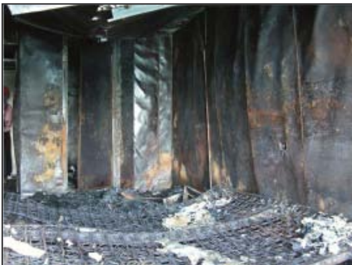
Figures 4a and 4b: The mist system was working properly in the stateroom above. The stateroom below is the only one where the mist system didn't work. USCG photos.
