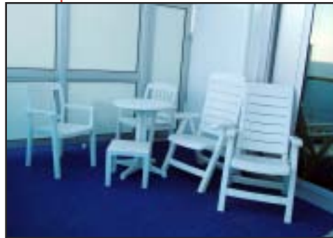
Figures 3a and 3b: Polycarbonate balcony partitions, plastic furniture, and polyurethane deck tiles before and after the fire. These materials were highly combustible and produced large quantities of very thick black smoke when burned. USCG photos.
