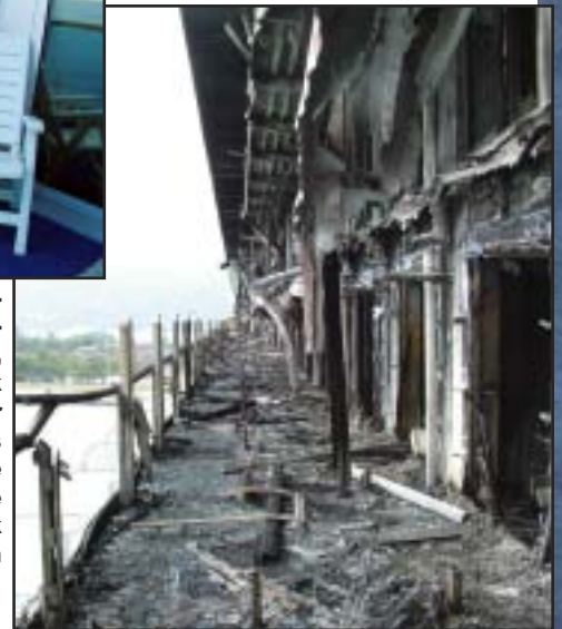
Figures 3a and 3b: Polycarbonate balcony partitions, plastic furniture, and polyurethane deck tiles before and after the fire. These materials were highly combustible and produced large quantities of very thick black smoke when burned. USCG photos.
