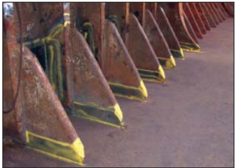
Figure 6b. Frames and toe brackets, after repair. USCG photo.
