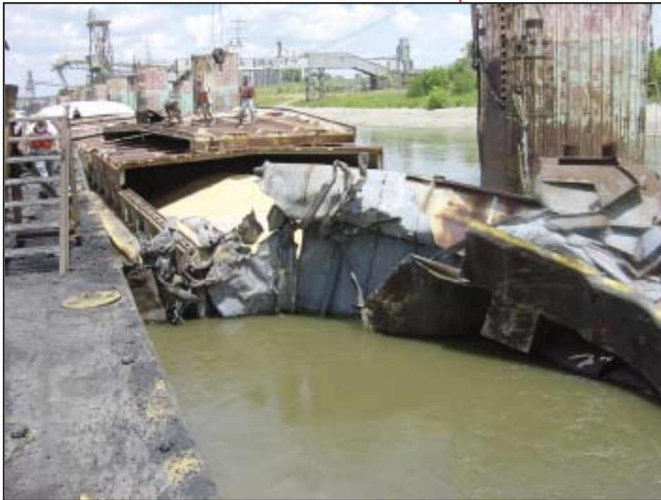
What's left of a hopper barge after an allision with the Eads Bridge on July 6, 2005. The vessel was traveling southbound on the upper Mississippi River at mile 179 as part of a 15-barge tow when it hit a bridge and broke away from the tow. USCG photos.
