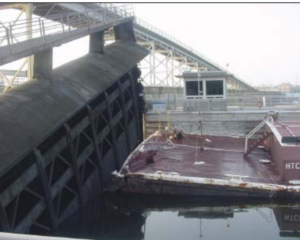
Figure 1: Barge HTCO-3016 pinned beneath the Wilson Lock/Dam upper main lock gate. USCG photo by CWO3 Tim Smith.
