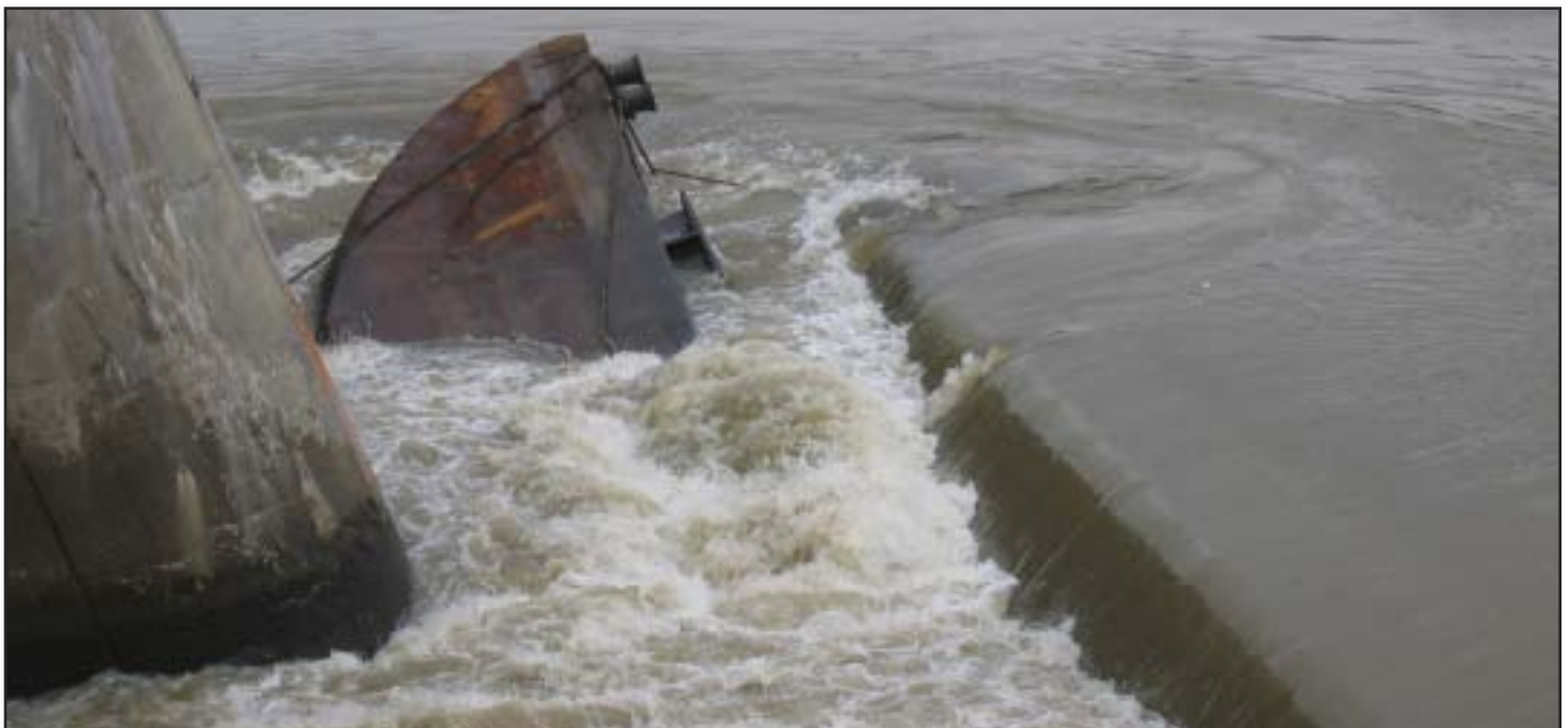
A sunken barge broken from the tow, jammed against the Montgomery Dam pier. USCG photo by LTJG Jesse Garrant.
