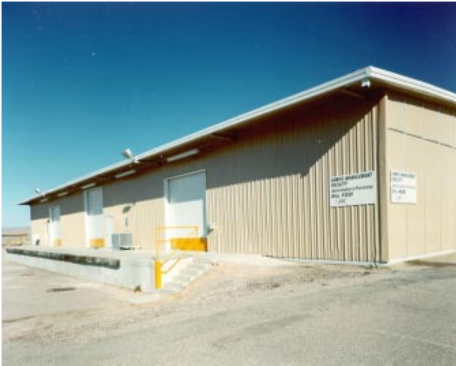
QA Sample Management Facility at Yucca Mountain
