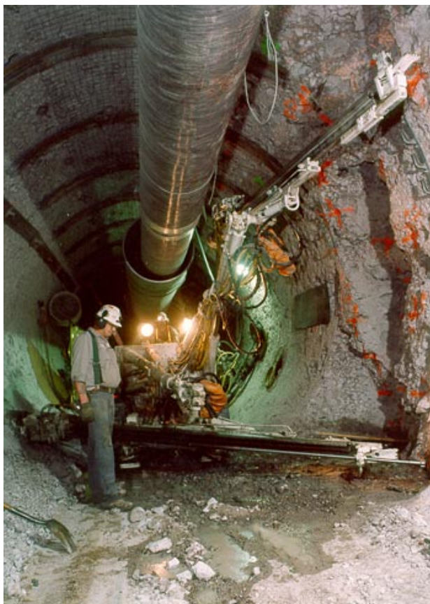
Drilling in Alcove 8
