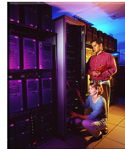
Supercomputer at an Office of Science user facility
