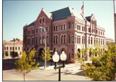
US District Courthouse, Sioux Falls, SD
