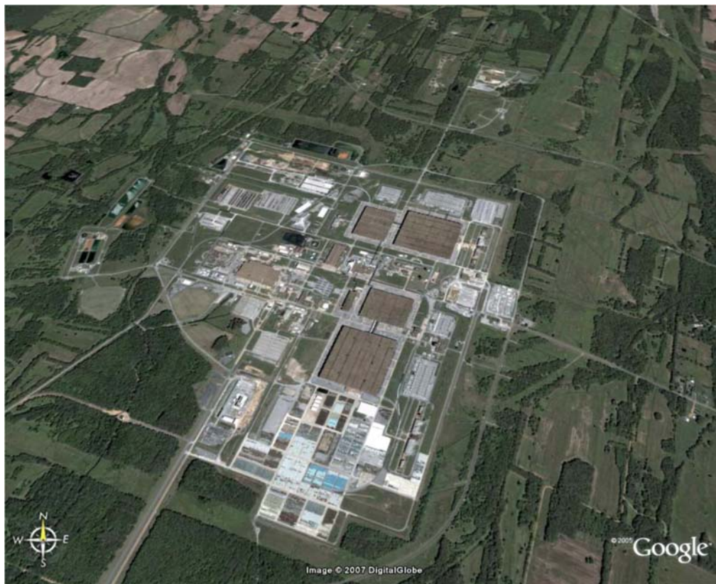
Paducah Gaseous Diffusion Plant (PGDP) Paducah KY
