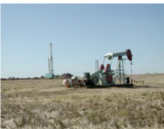
Carter Colliver #1 CO 2 injection well is shown in the background and the Colliver #13 producing well in the foreground, both part of the first CO 2 flood in Kansas.
