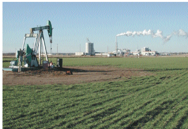
This pumpjack in Hall-Gurney oilfield, together with the ethanol plant in the background near Russell, KS, demonstrate the synergistic environmental and energy benefits of using industrial waste carbon dioxide in a CO 2 flood.
