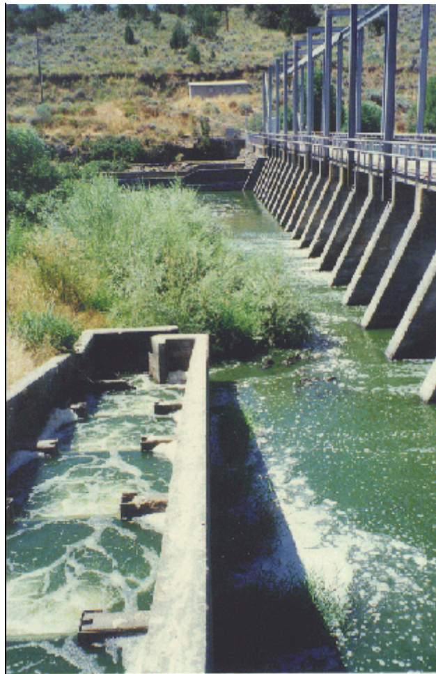
Figure 22 - View looking west along the cross channel from the existing fishway.
