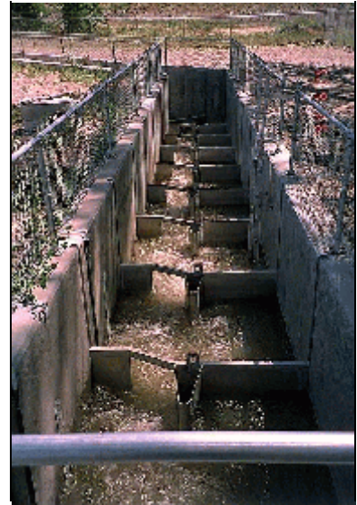
Figure 11 - View of the Redlands Fishway (looking downstream).
