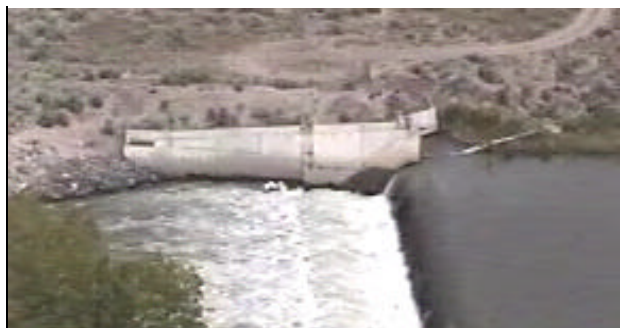
Figure 10 - View of Numana Dam vertical slot fishway.
