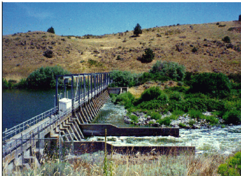
Figure 2 - Link River Dam looking east from Keno Canal.
