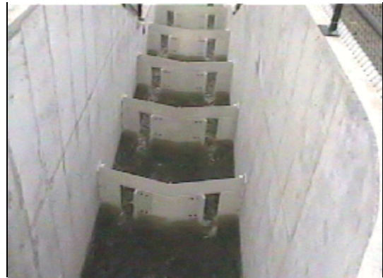
Figure 9 - Pyramid Lake Fishway exit ladder designed with chevron shaped vertical slot baffles (looking downstream).
