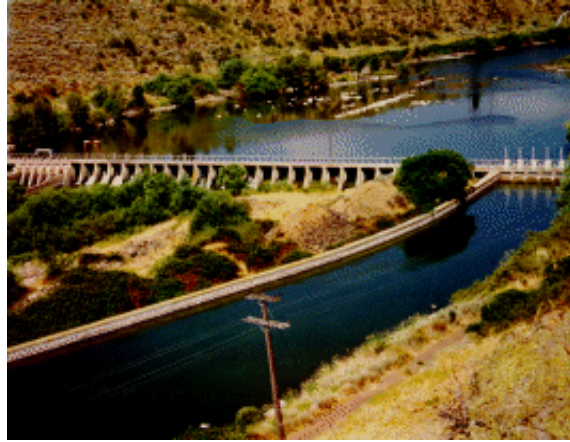
Figure 4 - View of the Ankeny canal and headworks.
