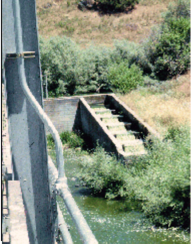
Figure 3 - View of existing Link River fishway.
