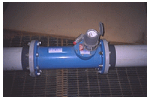
Figure 5. —Propeller flowmeter with analog output.
