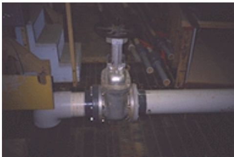
Figure 4. —Flow control valve.
