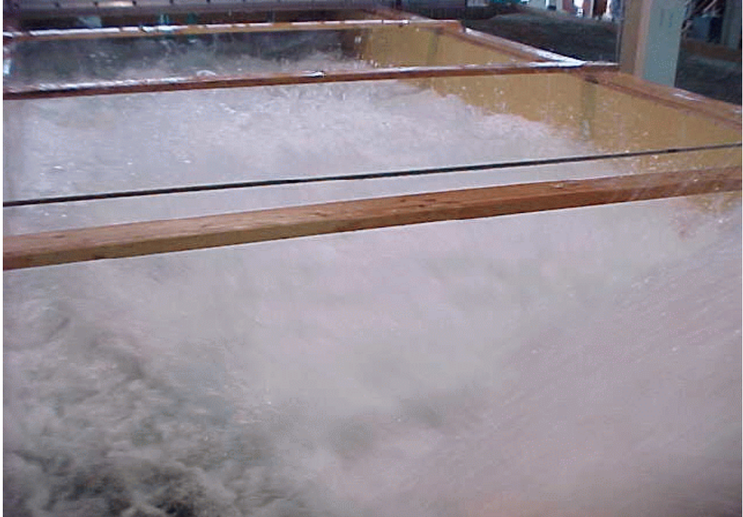
Figure 29. - Deflector Alternative with typical combined mid- and upper-outlet works operating. Reservoir at El. 1290 and high tailwater at El. 970.
