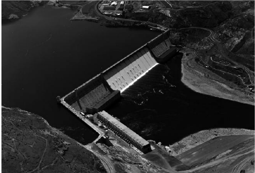
Figure 3. - Overall view of Grand Coulee Dam and Third Powerplant. Notice the north service yard adjacent to the Third Powerplant.
