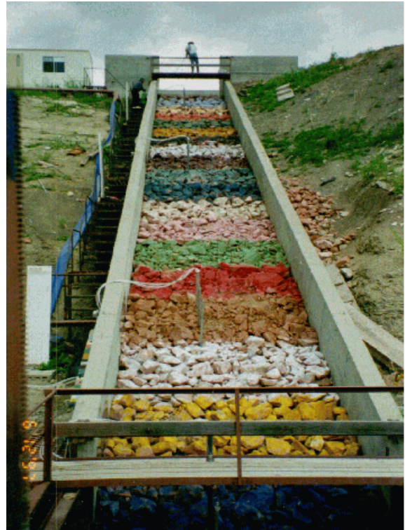
Figure 1. - Embankment overtopping research facility with riprap protection. Each 1.5 m wide band of rock was painted a different color to assist with observations of rock movement during the 1997 tests. (fig1.bmp)
