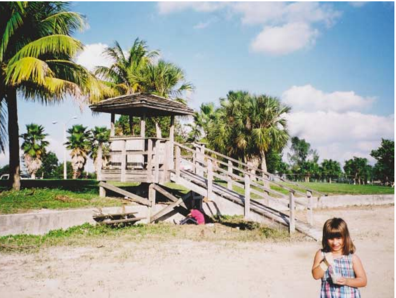
Under the boardwalk. University of Florida students measure arsenic under CCA-treated wood structures to gauge the extent to which the metal leaches from treated lumber. Although the chemicals in CCA are largely fixed in treated wood, problems arise when the lumber degrades or is burned at the end of its usefulness. The length of the service life of CCA-treated wood is debated, but most experts agree that an influx of the material will soon hit the waste stream.
