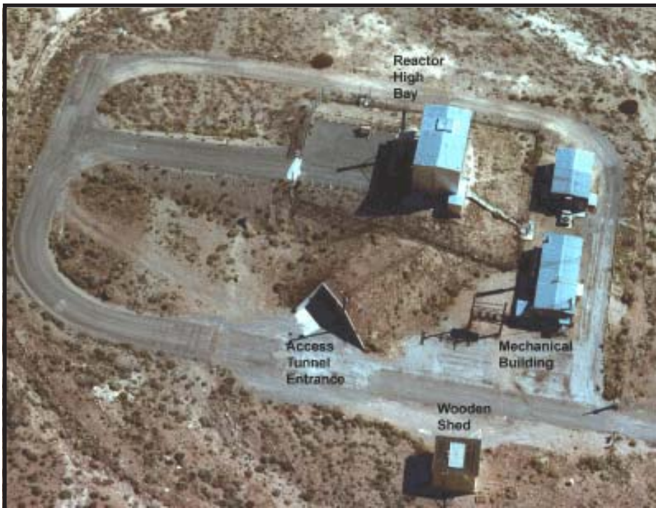
Aerial view of Super Kukla showing the Reactor High Bay, Mechanical Building, Access Tunnel Entrance and Wooden Shed.
