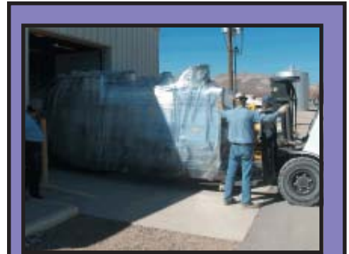
Workers remove the glovebox from the Visual Examination and Repackaging Building.
