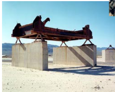
Rail Road Bridge
