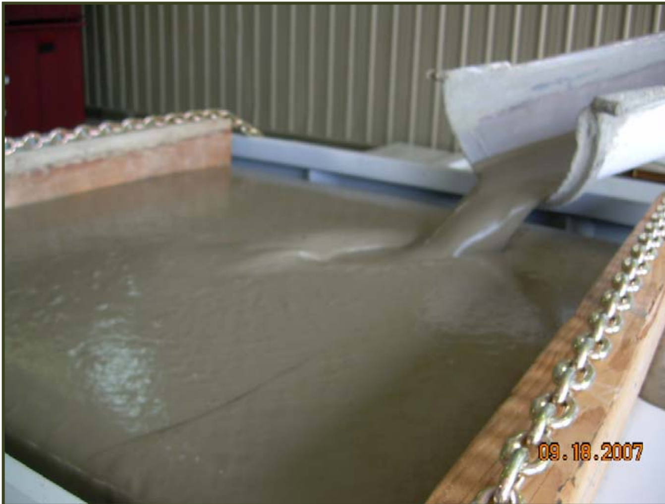
Mixed Waste Drums Encapsulated in a B-25
