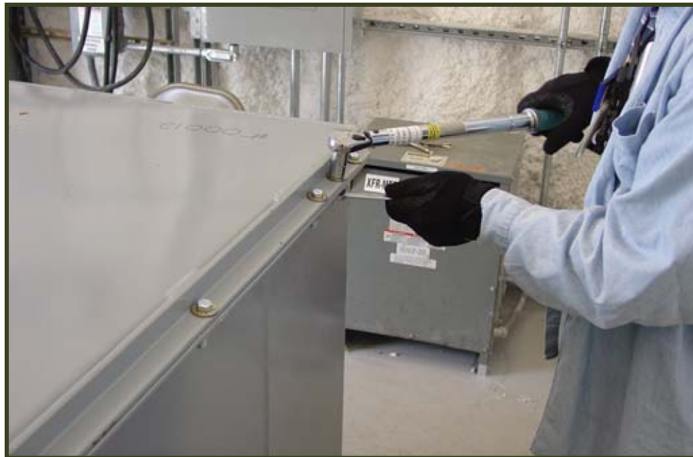
Steel lid bolted to container
