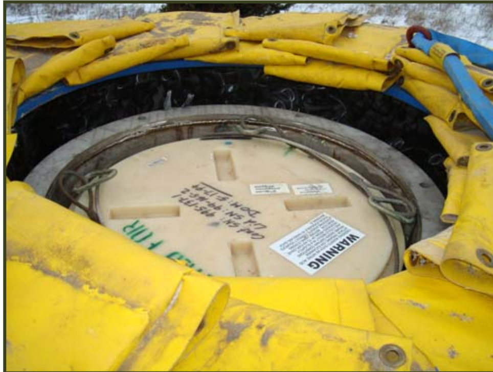
HIC placed in stainless steel overpack
