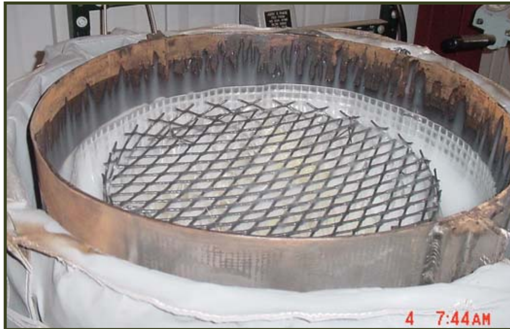
Debris waste placed into form
