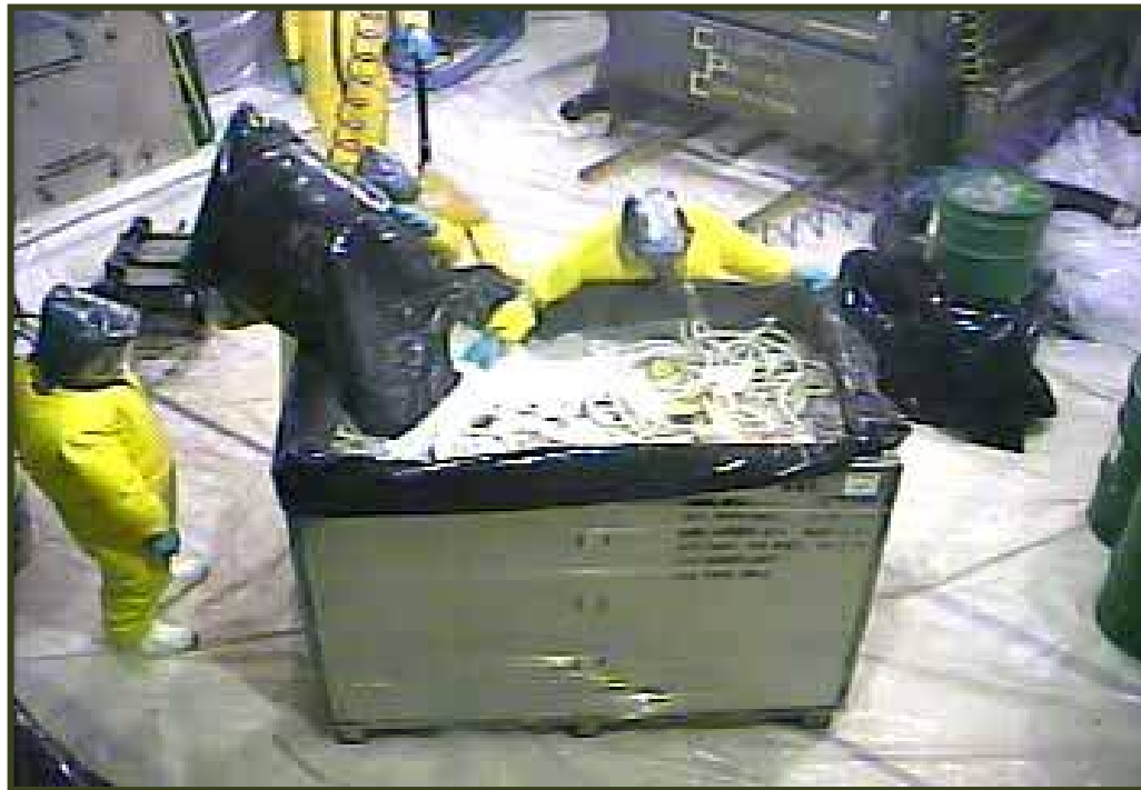
Loading debris into stainless steel box
