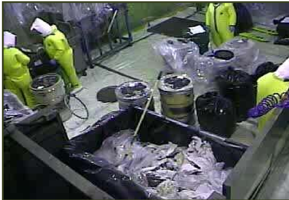
Loading debris into stainless steel box
