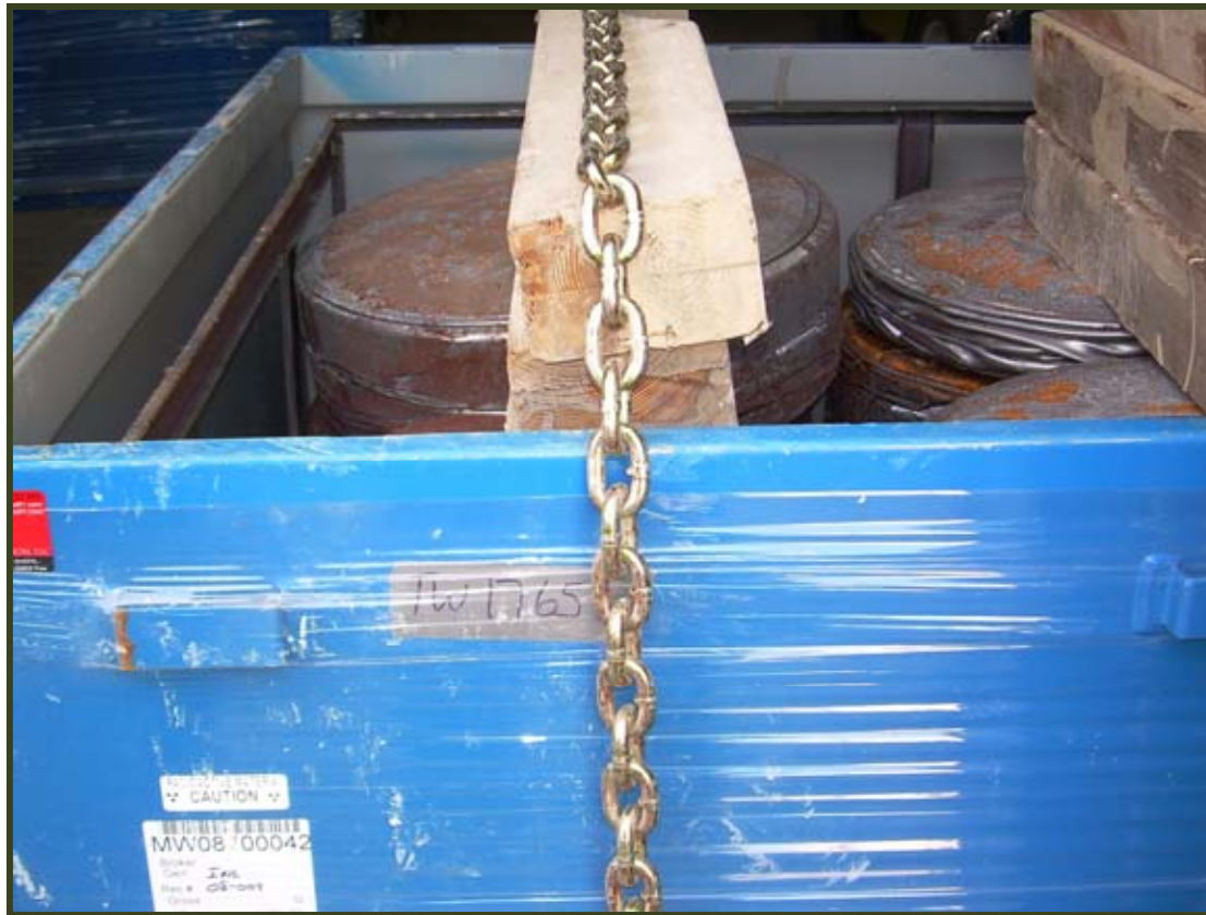
Debris waste prepared prior to pouring grout
