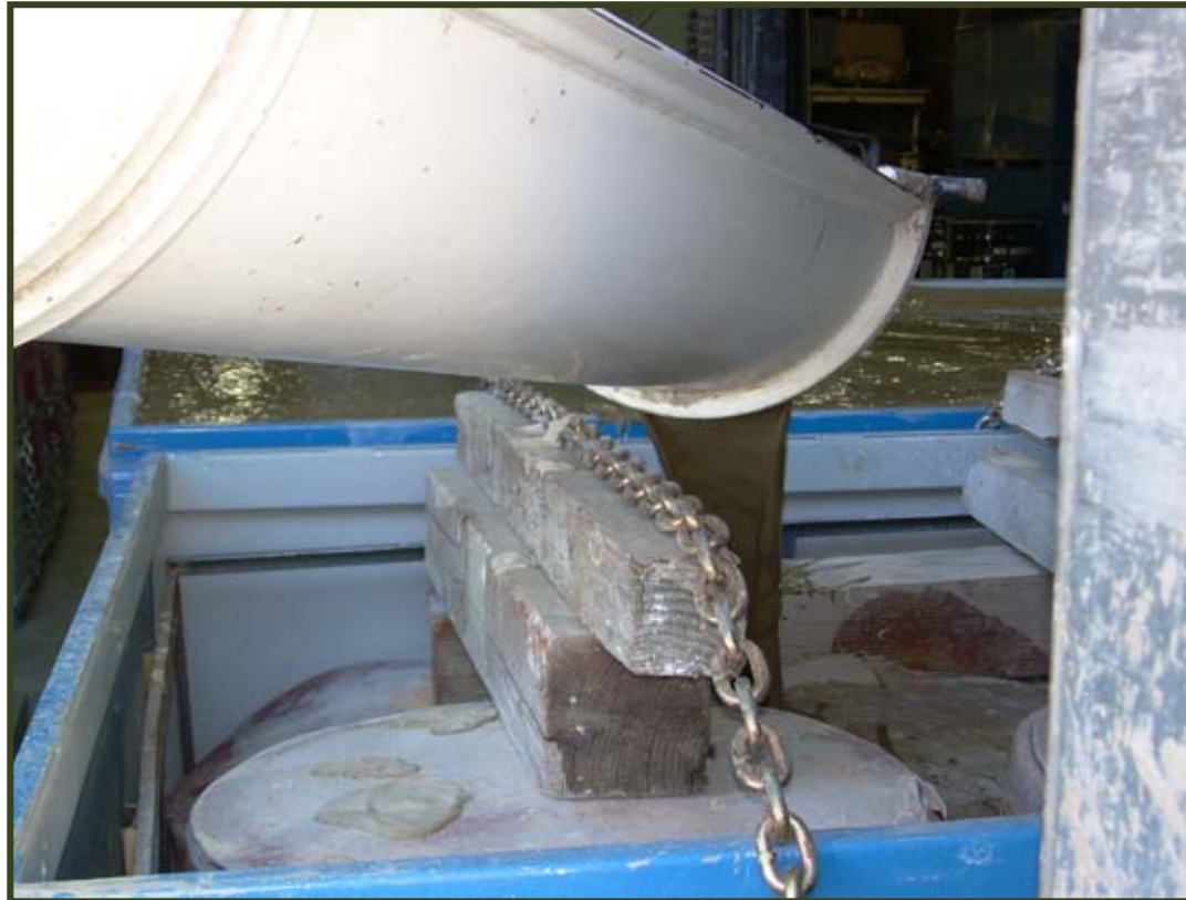
Grout poured around debris
