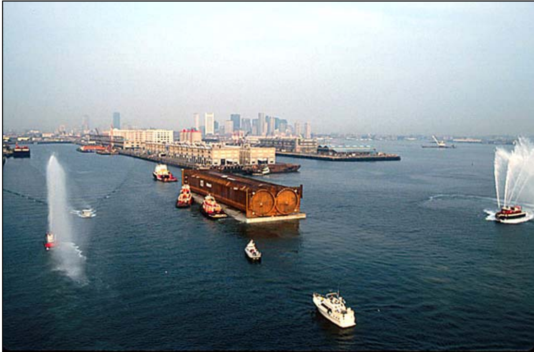
Figure M-3. Tube Sections for the Ted Williams Tunnel (excerpted from www.bigdig.com )
