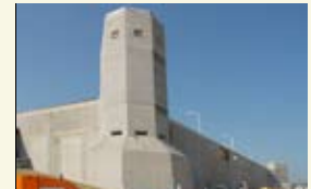
Highly Enriched Uranium Materials Facility, Y-12.
