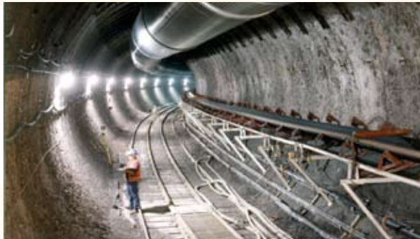
Exploratory Tunnel, Yucca Mountain.
