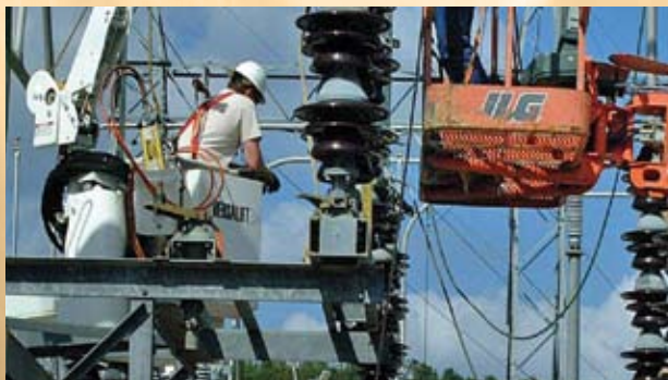
Substation Work, Southwestern Power Administration.
