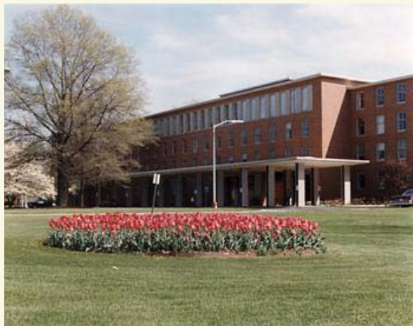
DOE, Germantown Complex
