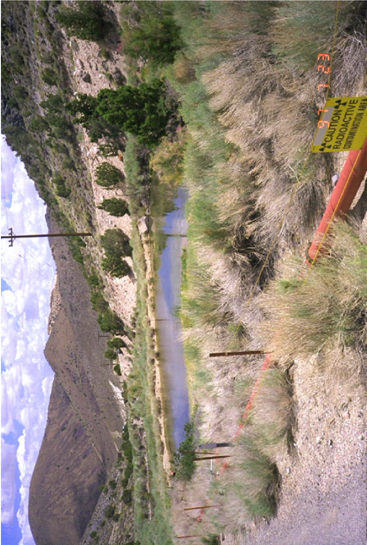
Figure 3.0 Photograph of E Tunnel Containment Ponds (07-23-97)
