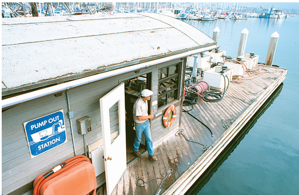
Sewage solution. Dockside pumpout stations are a far cleaner alternative to just dumping sewage overboard.
