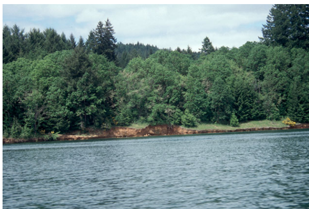
Photo 2-2. Shoreline erosion near Elks Picnic Area.
