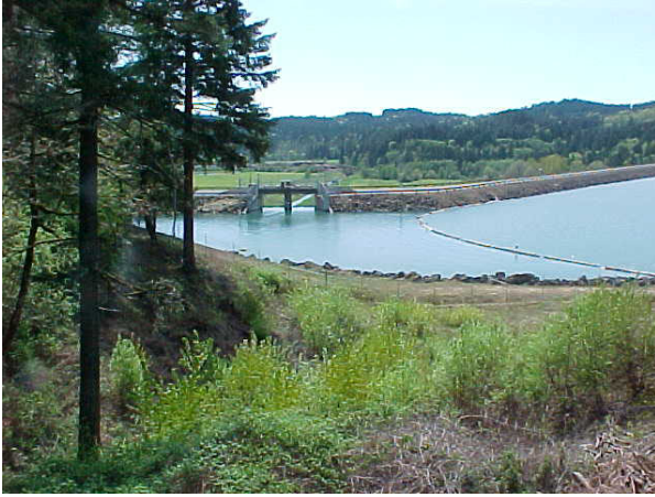
Photo 1-2. Scoggins Dam and spillway at full pool.
