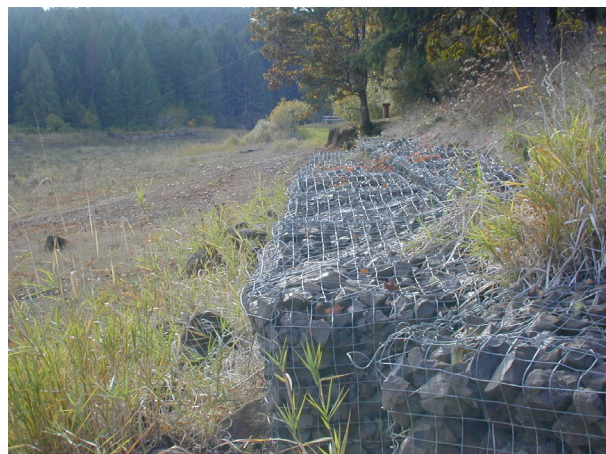
Photo 2-3. Shoreline erosion control structure at Sain Creek Picnic Area (at low pool).
