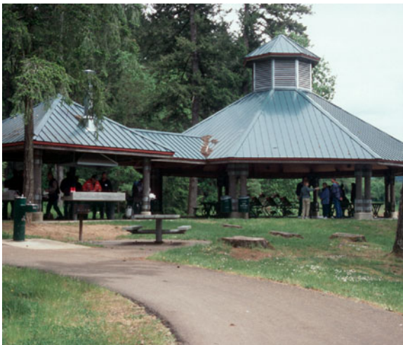
Photo 3-8. The Torvend Pavilion at Sain Creek Picnic Area.
