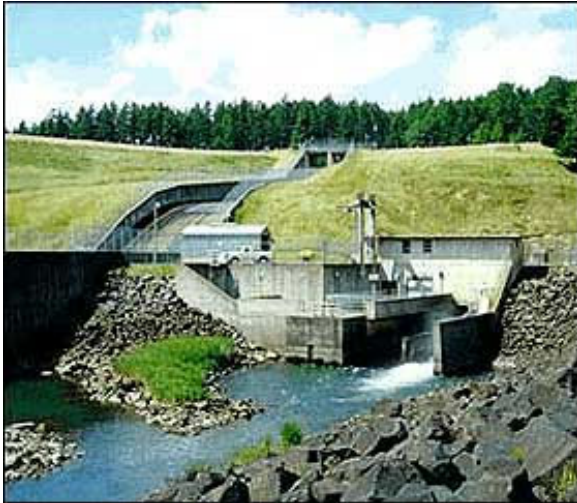
Photo 3-2. Scoggins Dam, spillway, and operations facilities below the dam.
