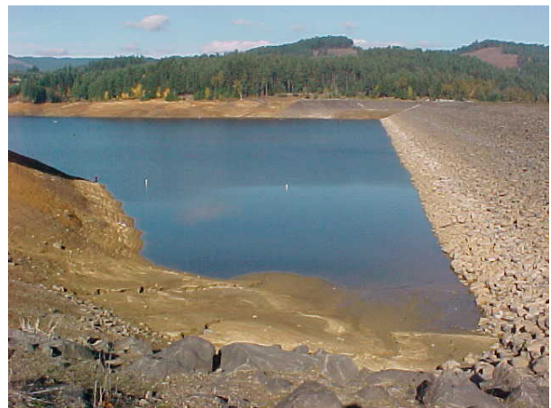
Photo 3-1. Scoggins Dam at low pool (October 2001).
