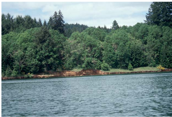
Photo 2-2. Shoreline erosion near Elks Picnic Area.
