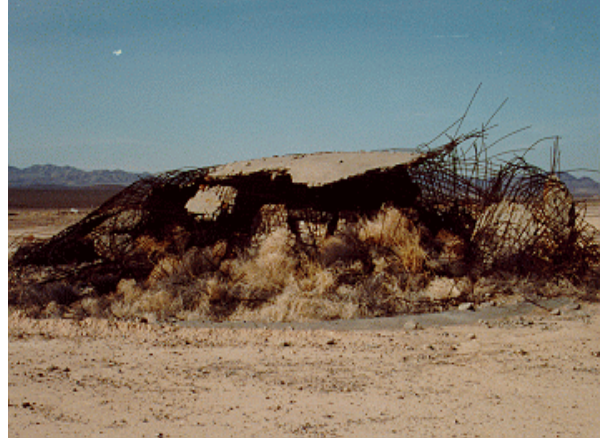
A collapsed six-inch thick concrete dome.
