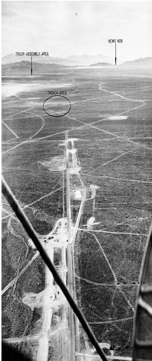
View from the top of the Smoky 700-foot tower, looking south.
