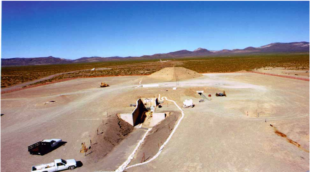
BEEF, showing the blast berm, which deflects blasts from high explosive detonations on the firing table to the front of the berm.
