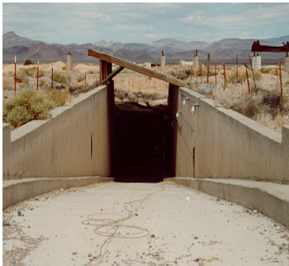
Garage/shelter entrance as it appears today.
