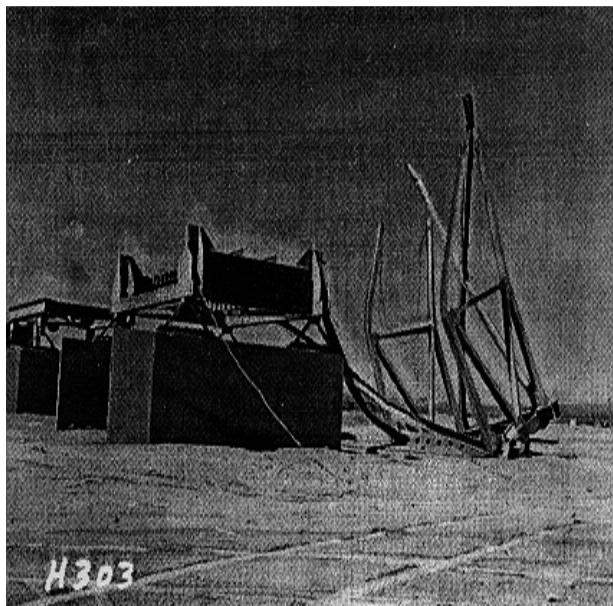
Open frames structure after the Encore test.
