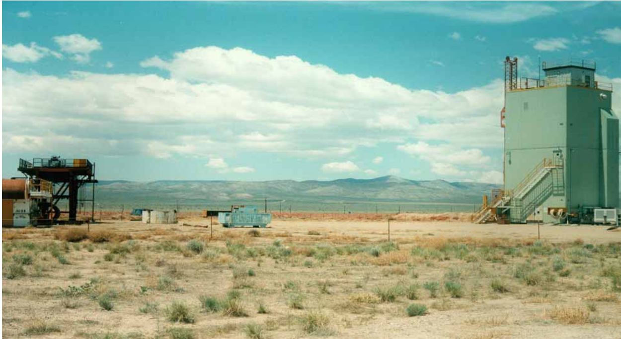
Fortune Training Tower located to the west of Tweezer Road in Area 6.
