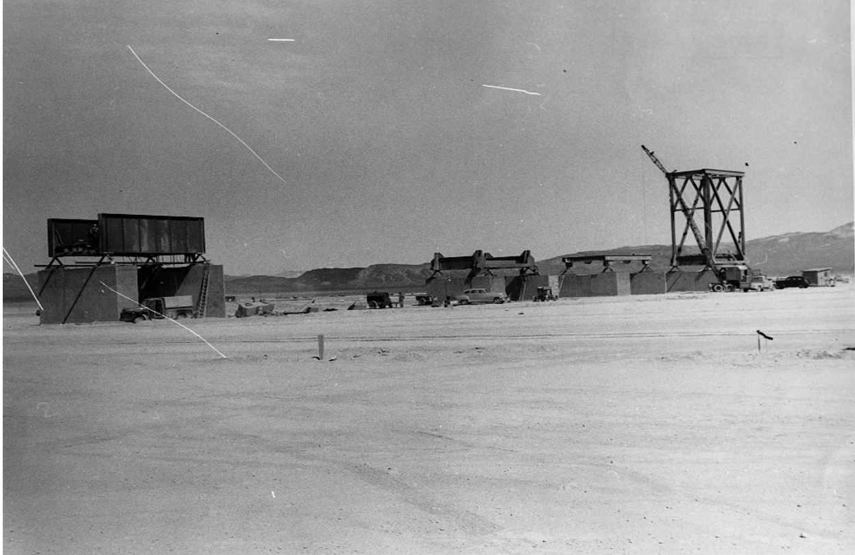
Four open frames structures are readied for the Encore test. The single-track railway bridge at the far left still remains today, minus its upper framework. The structure was 2,200 feet from the Encore ground zero.
