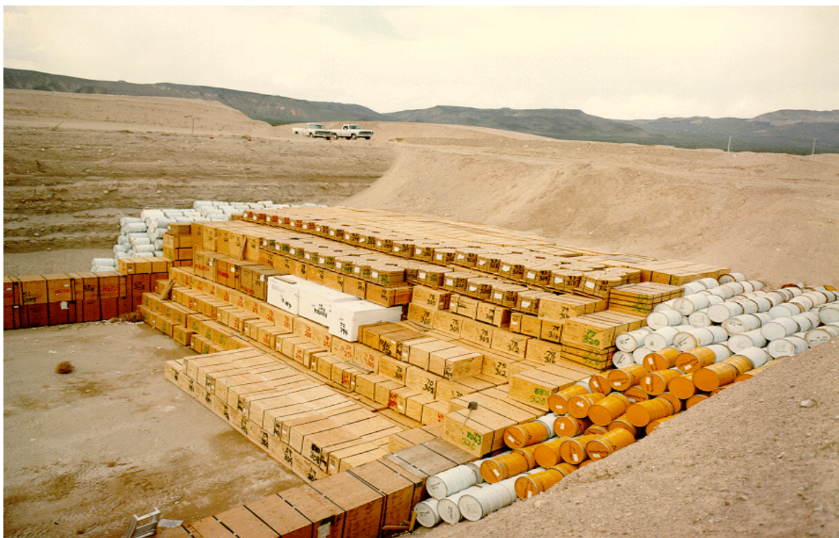
A typical low-level radioactive waste storage pit.
