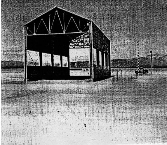
A drag type Butler building prior to the April 1955 MET (Military Effects Test).
