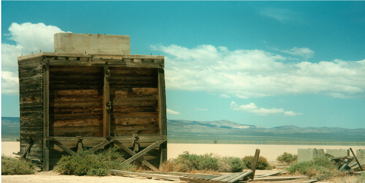
One of three camera towers built by Sandia National Laboratories to photograph inert bomb (non-nuclear) drops at Yucca Lake in Area 6.
