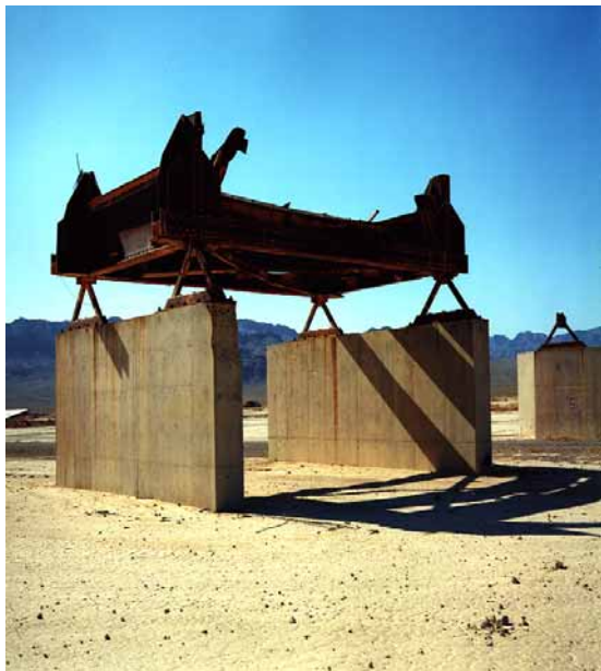
Open frames structure today.
