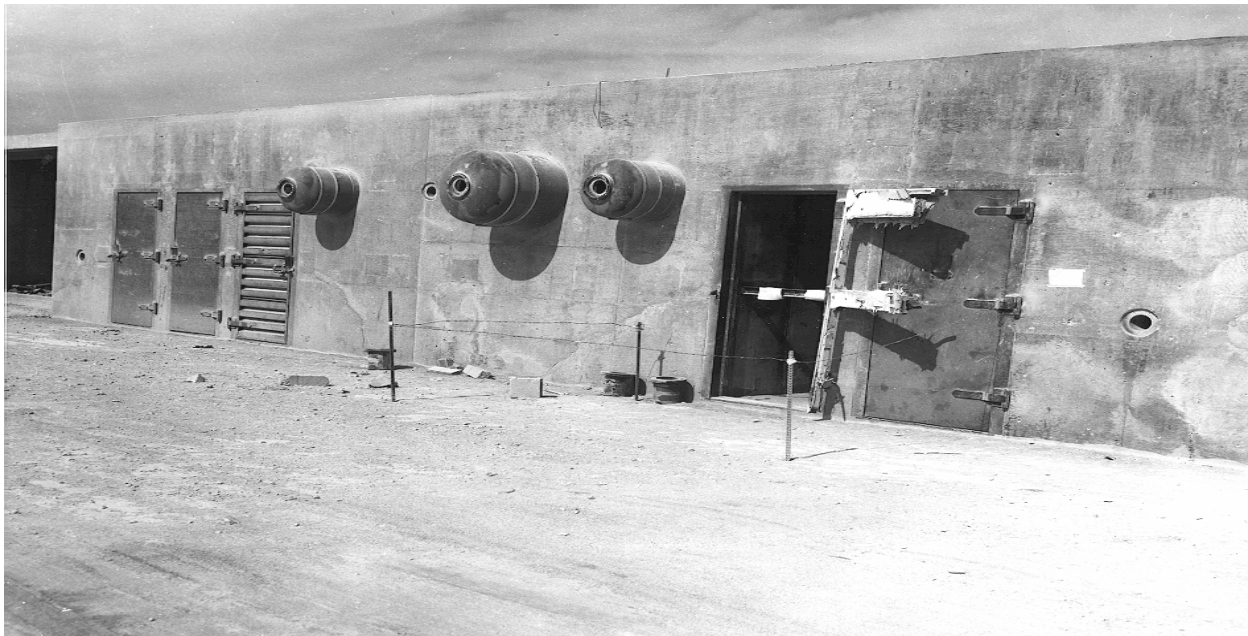
One of the industrial buildings (motels) shortly after it was exposed to the 1953 Encore test.
