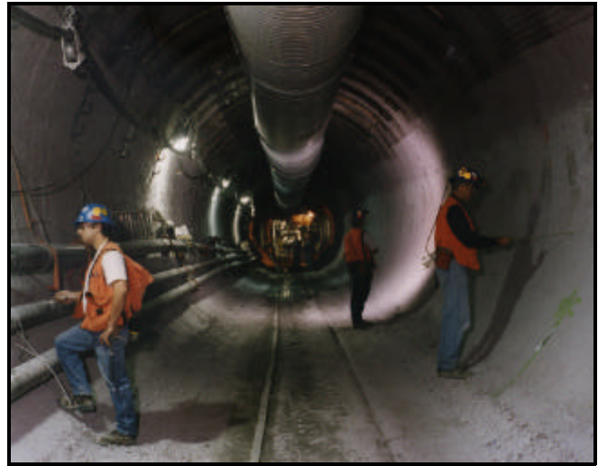
Yucca Mountain Tunnel
