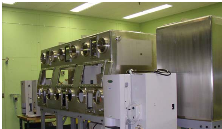
Installation of new LECO instrument at CMR Wing-7
