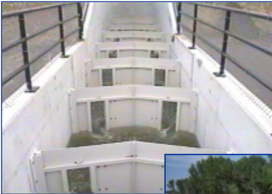
Concrete Flume and Baffle Fishway
