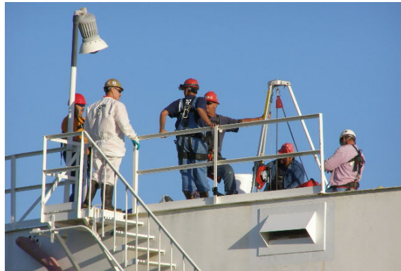
SPR's personnel prepare to inspect Bryan Mound's BMT-3 crude oil tank.
