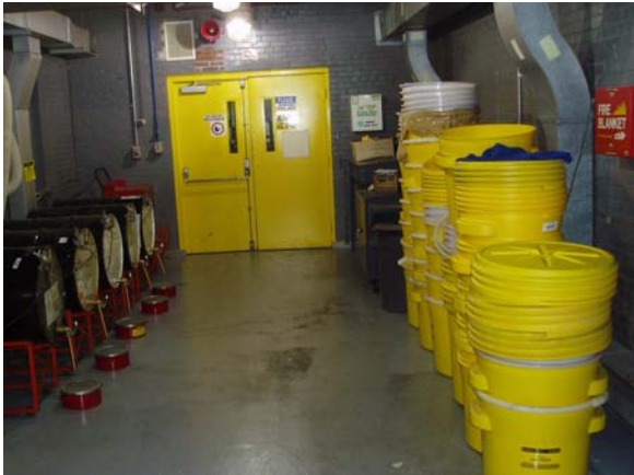
An interior view of the refurbished Chemical Handling Facility at NETL-Pittsburgh.
