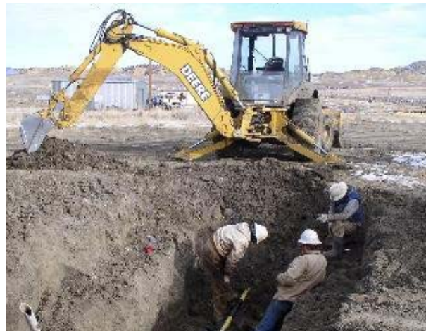
RMOTC employees Rick McLaughlin, Darwin Hoffer, and Kevin Greene prepare to replace a flowline at well 56 Lx 3.
