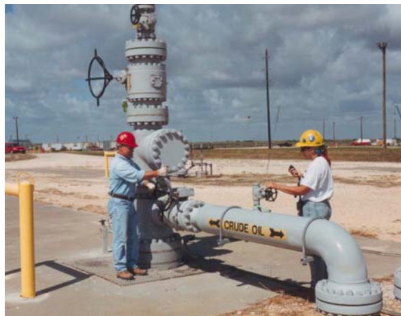
SPR employees working at a Bryan Mound wellhead.
