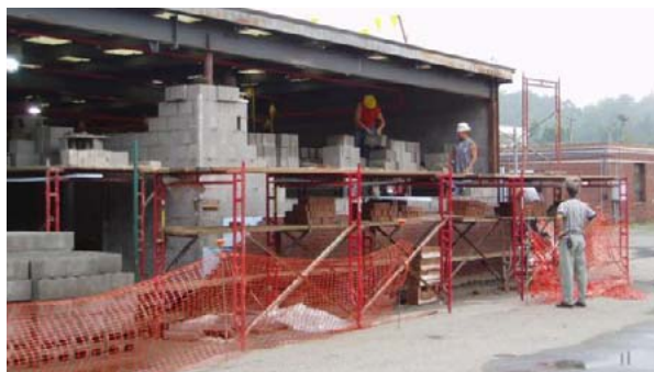
Renovations to NETL Pittsburgh’s Chemical Handling Facility.
