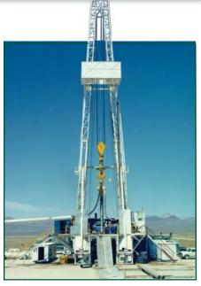
Wells are drilled to collect groundwater samples, aiding scientists in determining contaminant boundaries and movement.
