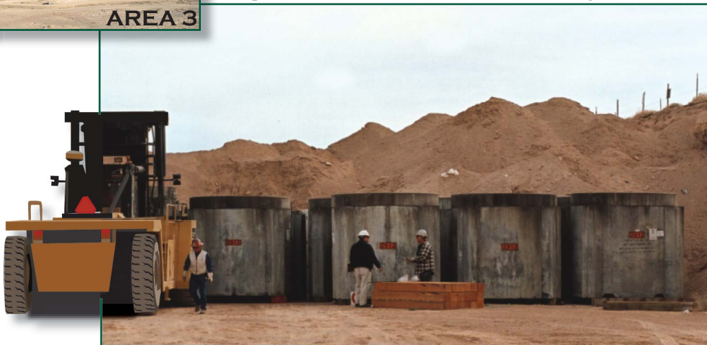
Concrete monoliths of low-level radioactive waste are positioned in a disposal cell at the Area 3 Radioactive Waste Management Site.
