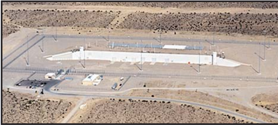
In addition to its physical isolation, two gun turrets at either end of the facility provide extended security at the DAF.
