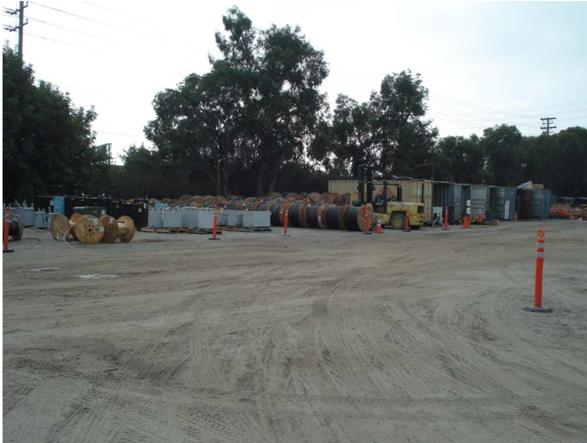
Figure 8: Looking east from center of peaker site.
