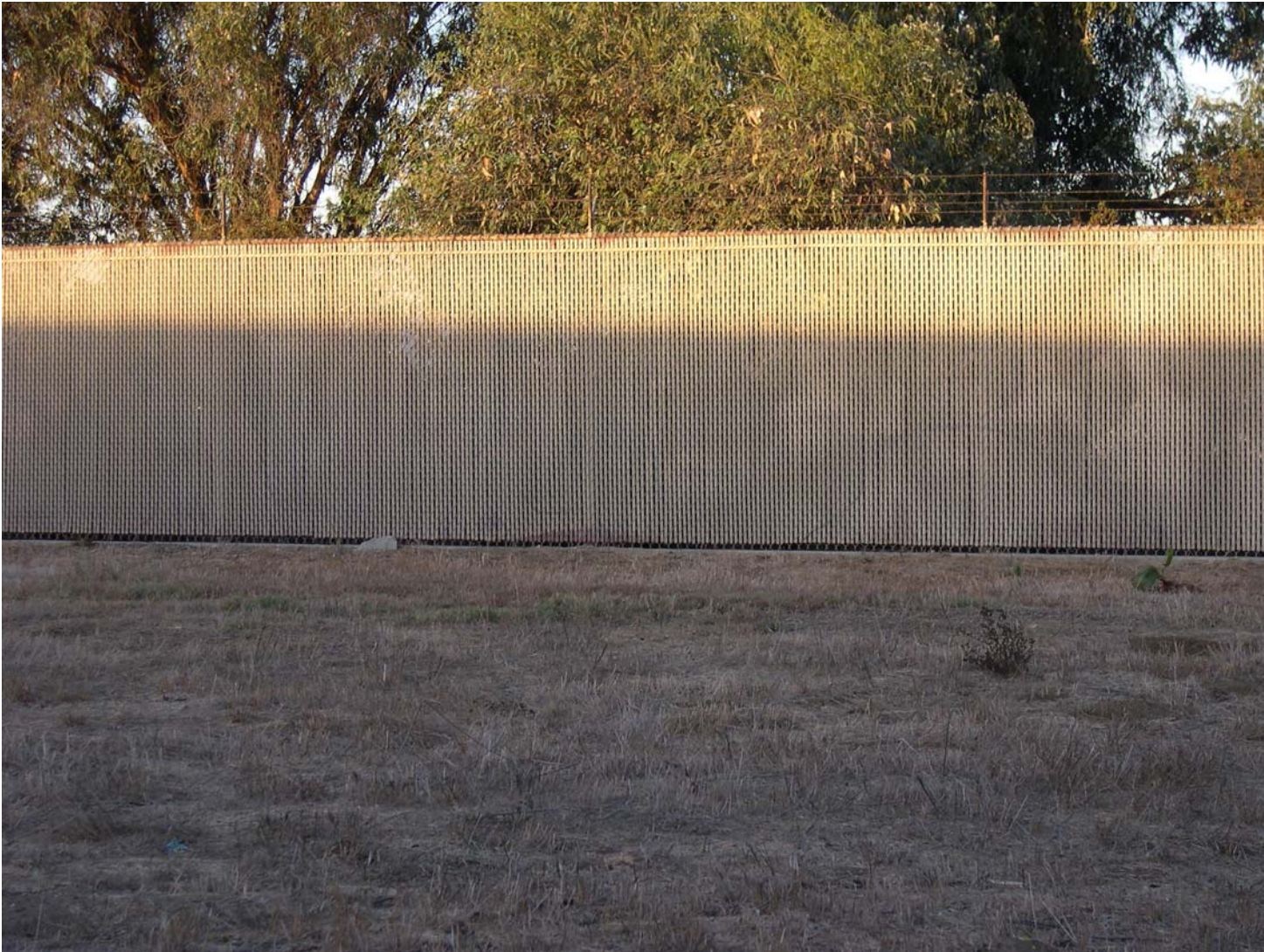
Figure 14: Looking west from Dumont Ave. at proposed site for access road.
