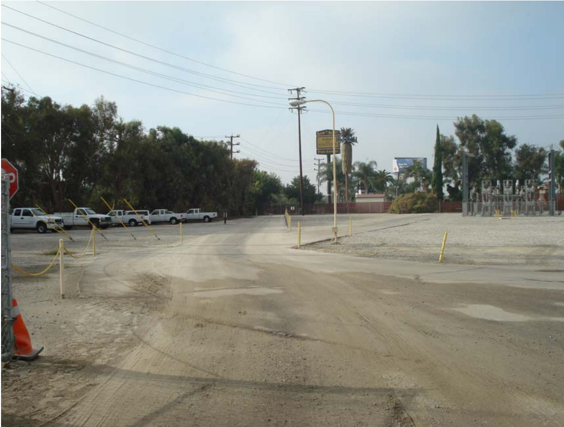
Figure 11: Looking south from center of substation at existing paved access.
